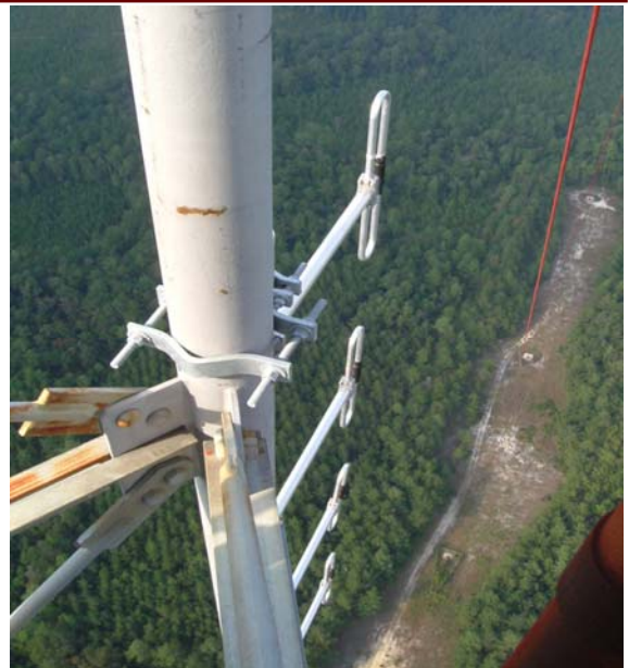
At 965 feet above ground, the CARES Wilmington repeater transmit antenna provides excellent signal coverage.
